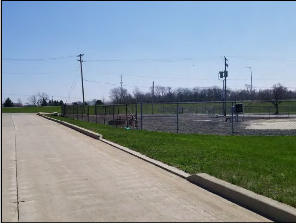
Figure 7 Photo of properties to the east of the subject property on Cabintown Road with an existing six-foot fence in the front yard.
