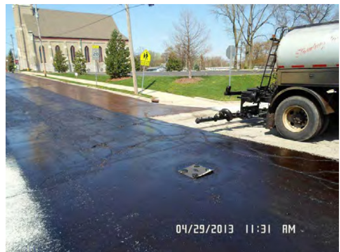
Figure 9 – CRF just applied to north side of Jackson Street. South side has cured to black color after 15 minutes. Lime screenings on Oak Street are visible on left side of picture.
