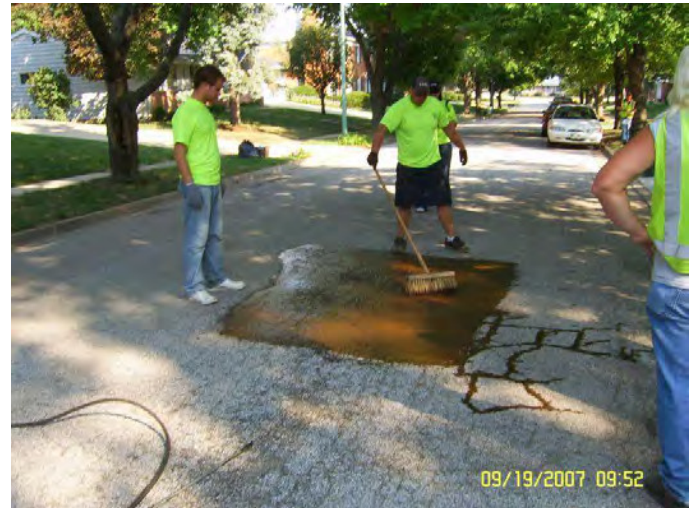
Figure 2 - CRF applied by hand applicator then broom finish
