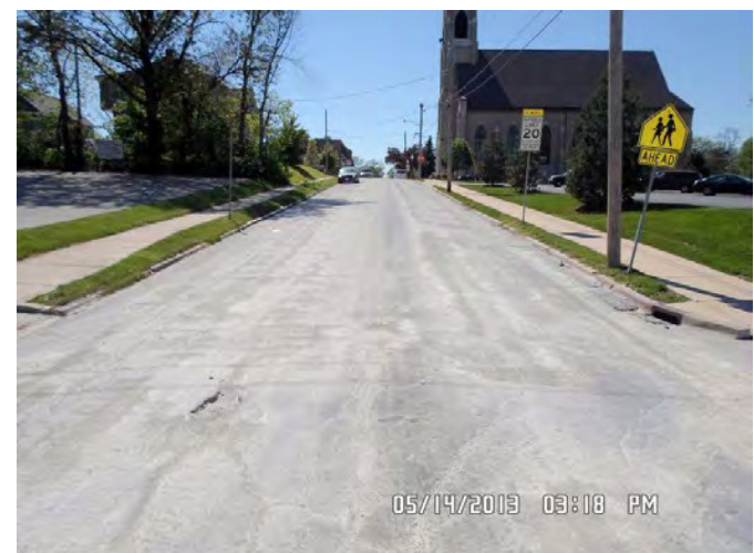
Figure 10- Jackson Street 9 days after CRF treatment
