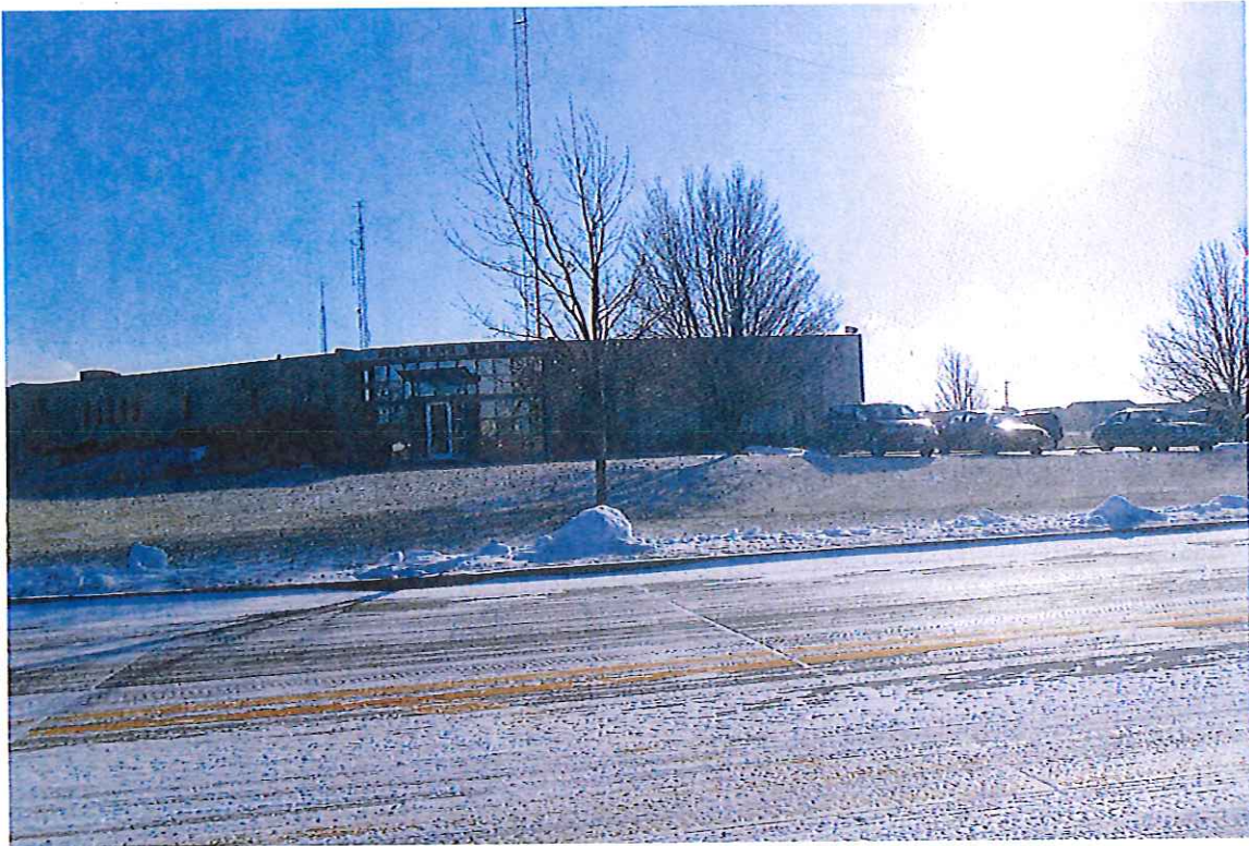
EAST VIEW ACROSS GREENWOOD
