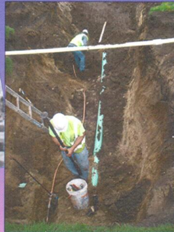
Crews replacing sewer & water services
