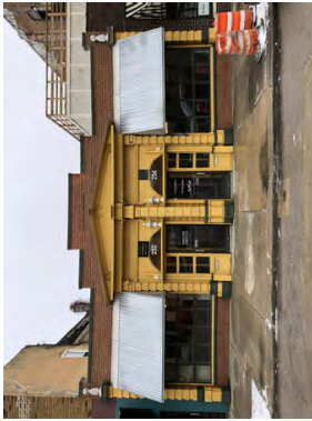
OVERALL VIEW OF EXISTING WOOD CLADDING FACADE WITH ORIGINAL FACE BRICK BEYOND.
