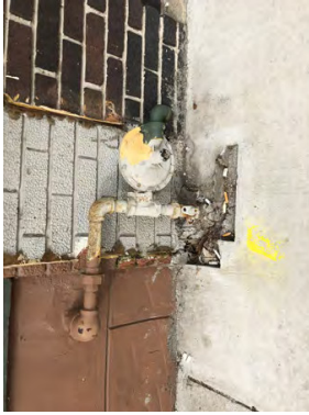
EXISTING GAS REGULATOR EXPOSED DURING INVESTIGATIVE DEMOLITION. SIDEWALK TO BE REPLACED.
