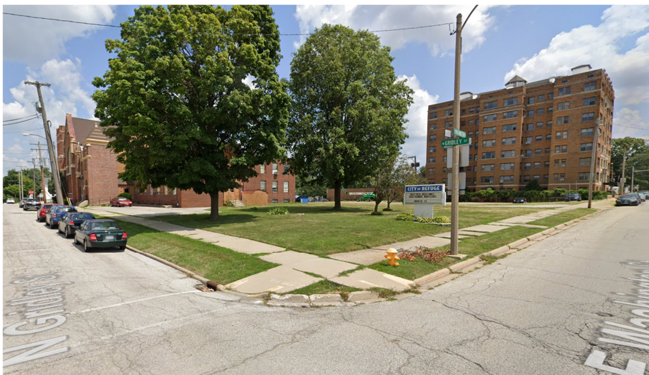
Attachment 3 - Ground-Level View
