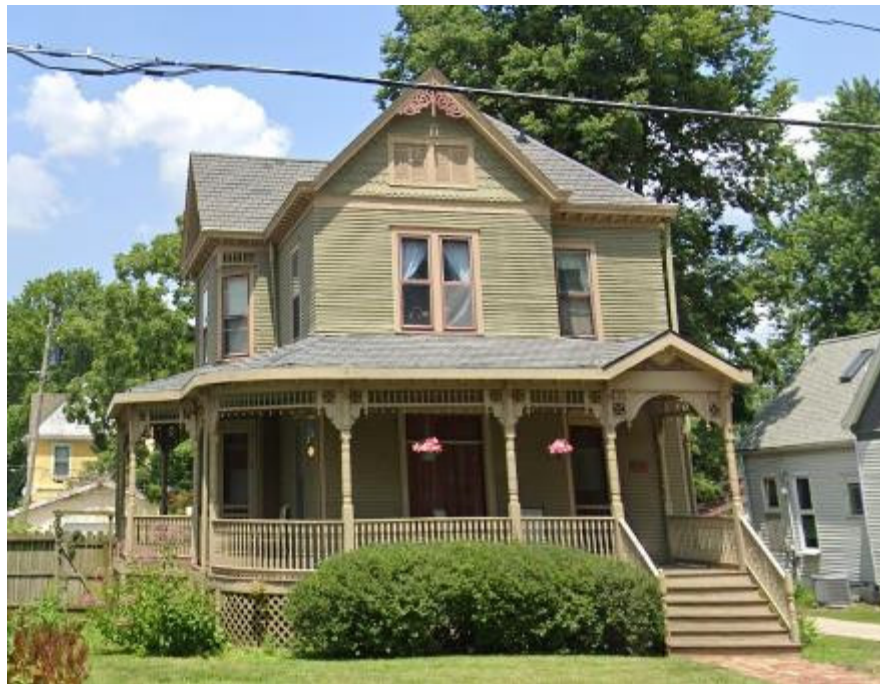
The subject property at 1212 E. Washington Street.
