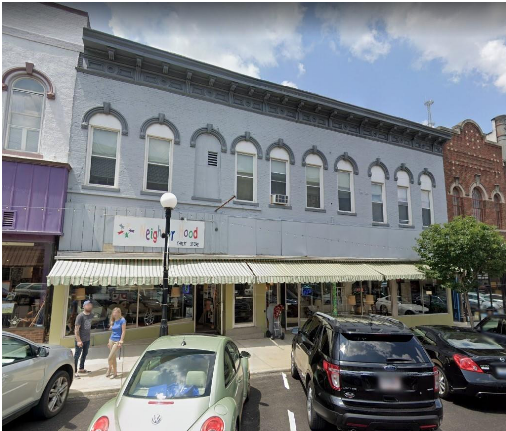
Above: The subject property at 406-410 N Main Street.
