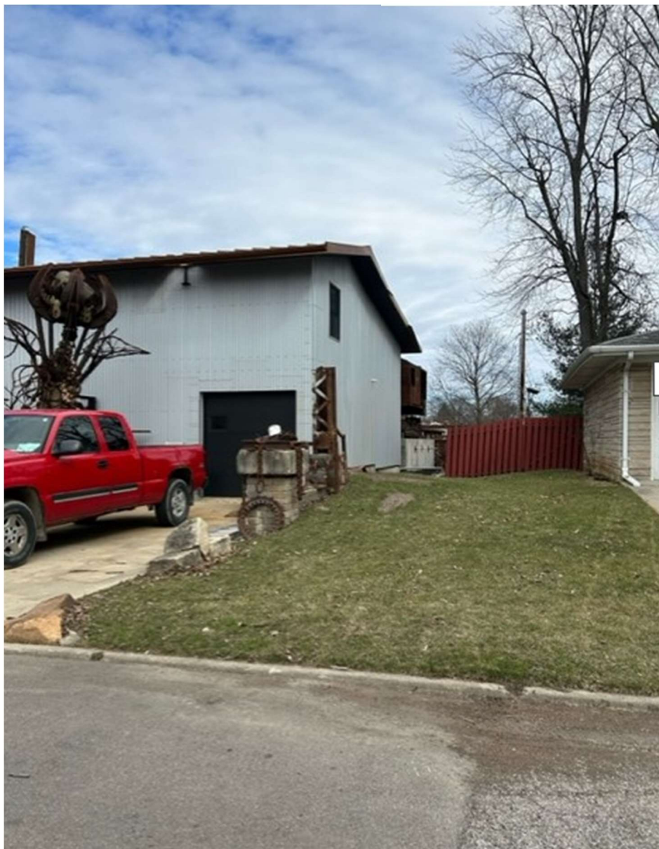
Attachment 3 - Ground-Level View (from Arlene Drive)
