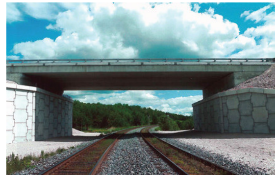
Example of a similar-looking bridge Source: Precast Solutions Article, Sprint 2011 Issue
