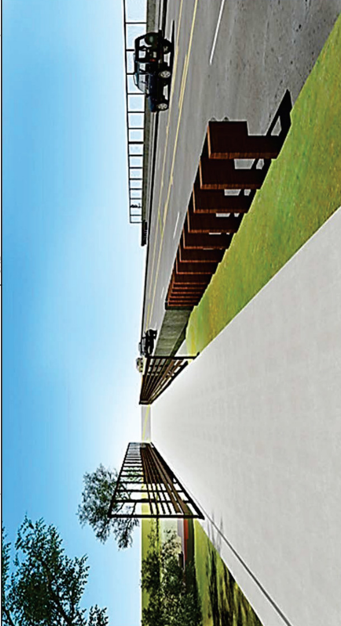
Five lane bridge 6-foot sidewalk on south; 2 nd bridge with 12-foot shared path on north side.
