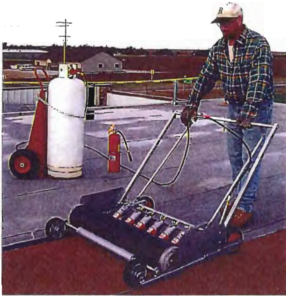
Portable cylinders on roofs are not prohibited by Section 6104.3.1. (Courtesy of Midwest Roofing Contractors Association, Glenview, IL)
