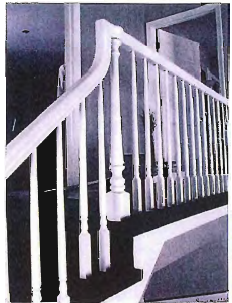
Transition from handrail to guard
