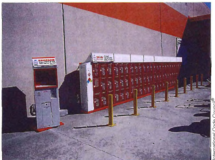
Automated cylinder exchange station
