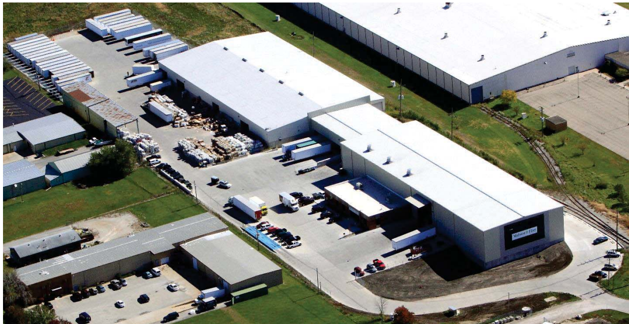
Midwest Fiber Recycling, Normal, IL - Material Recovery Facility
