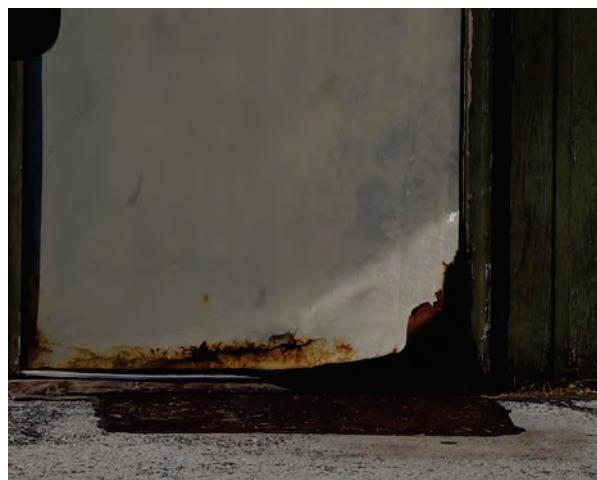
Left: Water seeping through the foundation wall of the boiler room at Bloomington High School. (1200 East Locust Street)
