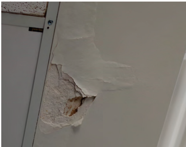
Left: Water damage on the interior of Bloomington High School. (1200 East Locust Street)
