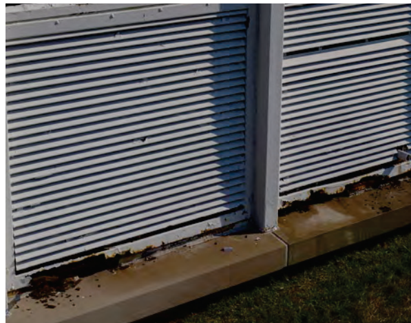
Right: The windows sills at Bloomington High School are rusted and deteriorated. (1200 East Locust Street)
