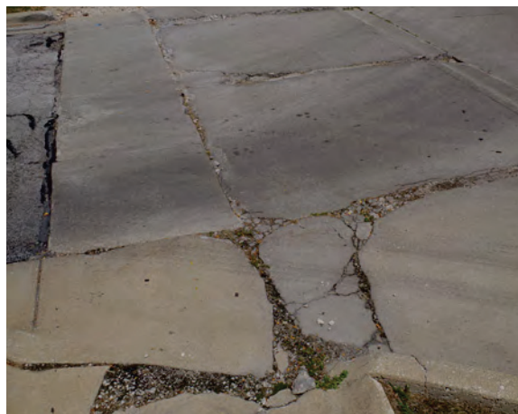
Right: The apron leading from IAA Drive to the eastern entrance Colonial Plaza is severely deteriorated.
