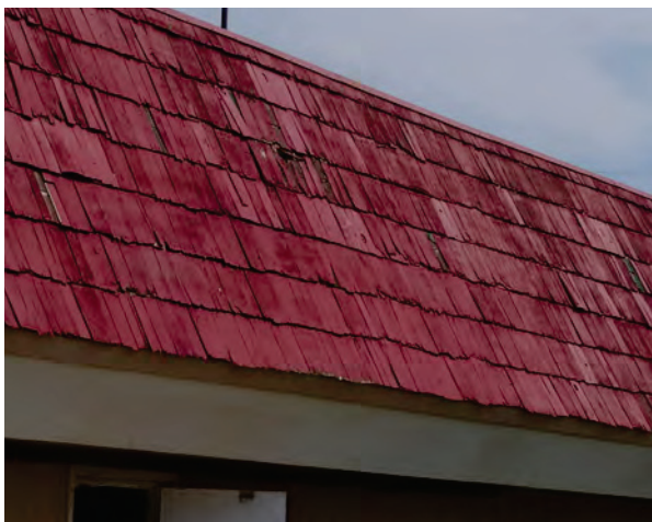
Left & Right: Deteriorated wood shingles on the roof of Kep's Country Kitchen. (506 IAA Drive)
