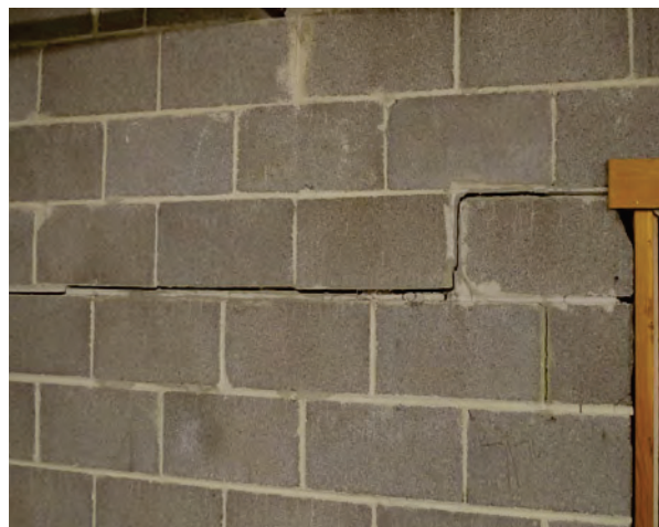
Left & Right: Cracking in the concrete block walls of the former K--Mart. (1608 East Empire Street)
