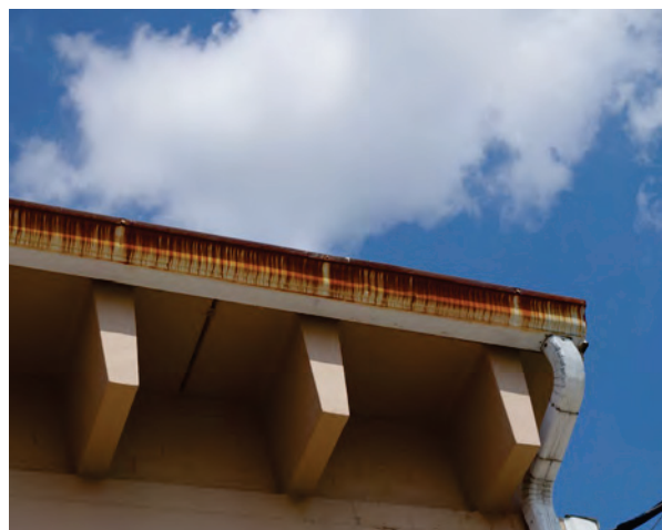
Right: Rust from the roof of the Community Players Theatre is staining the gutters. (201 Robinhood Lane)
