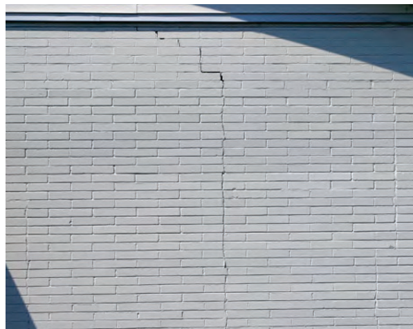
Right: Cracking in the exterior brick wall of this multi-tenant building. (1328 East Empire Street)
