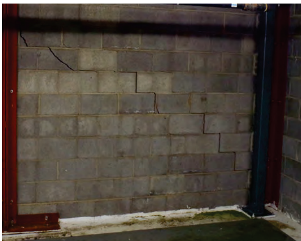
Left & Right: Cracking in the concrete block walls of the former K--Mart. (1608 East Empire Street)
