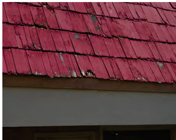
Left & Right: Deteriorated wood shingles on the roof of Kep's Country Kitchen. (506 IAA Drive)
