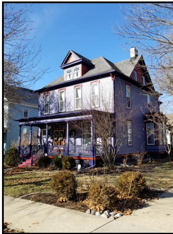
Figure 1 Photo taken 1/16/2020 of the existing roof.
