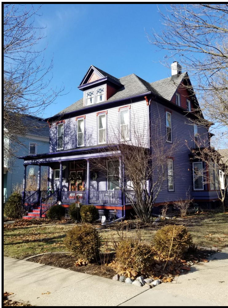
Figure 1 Photo taken 1/16/2020 of the existing roof.
