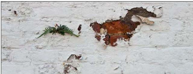
The peeling paint is likely incompatible with the brick or may be caused by moisture. The plant growth indicates moisture trapped in the wall. The paint should be removed.
