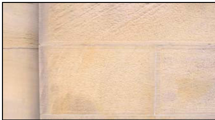
Limestone – A sedimentary rock; used for building walls, window sills and lintels, ornamental stone trim, sculpture and for producing lime.
