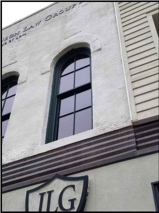
Figure 7 Window at 115 W. Front Street.
