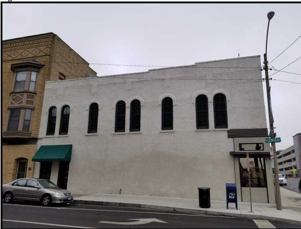
Figure 8 West elevation of 115 W. Front Street.
