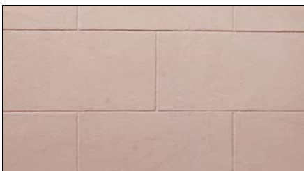
Scored Stucco – Smooth finish with scoring to simulate stone joints.
