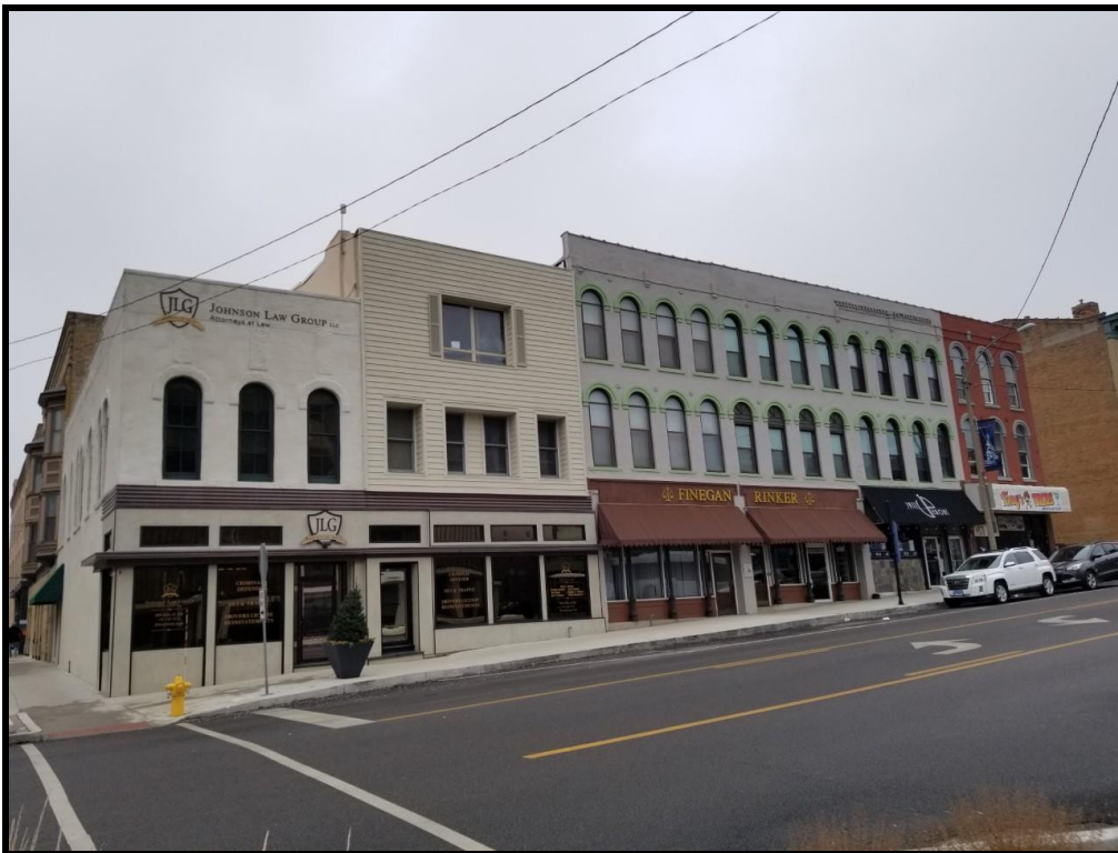
Figure 4 111-115 W. Front Street Streetfront facades
