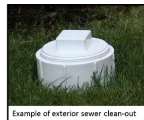
Example of exterior sewer clean-out
