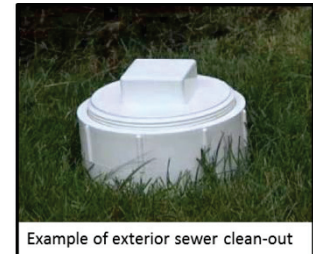
Example of exterior sewer clean-out
