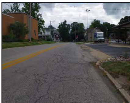
Above: The pavement along North McLean Street is deteriorated.
