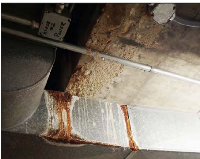
The HVAC duct work and concrete reinforcing in the basement of the former bank have rusted due to moisture infiltrating the concrete.
