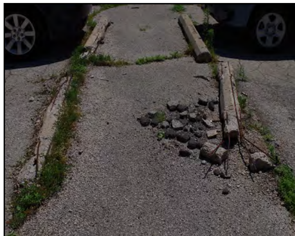
Right: The parking stops at 500 East Jefferson are crumbling and deteriorated.
