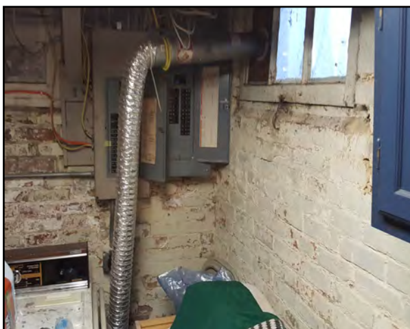
Left: Flexible exhaust venting ran to the window of the salon presents a carbon monoxide hazard.
