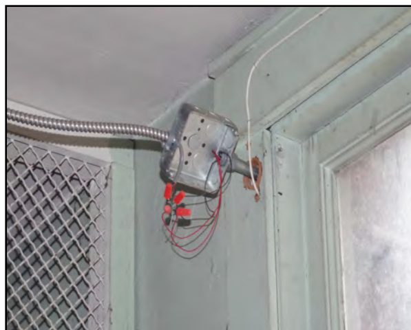
Left & Right: Open electrical junction boxes with exposed wires located throughout the school.
