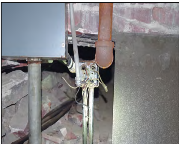
Left & Right: Open electrical junction boxes with exposed wires located throughout the school.
