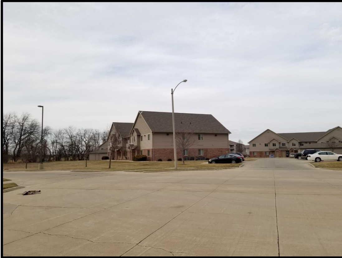
Figure 7 Multi-family residences at 2304 Gerig Drive.
