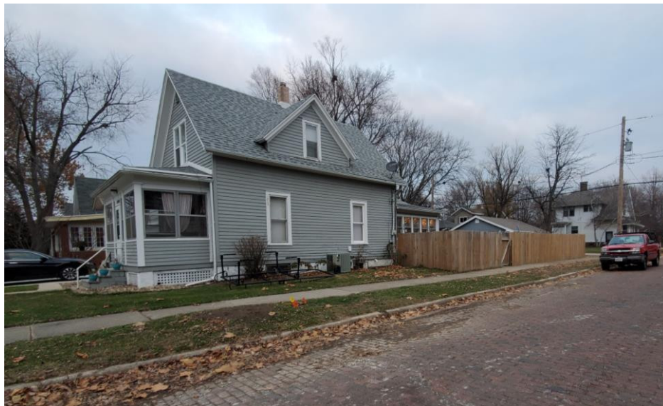
Figure 3: A side view of the subject property
