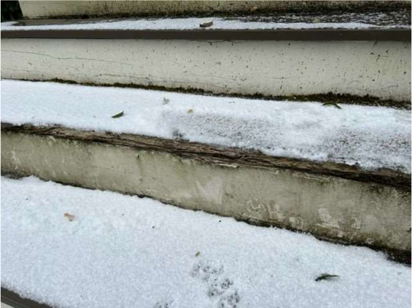
Main Porch Stairs
