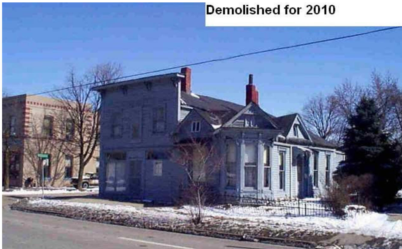
Attachment 1: Image of “protected structure” prior to demolition
