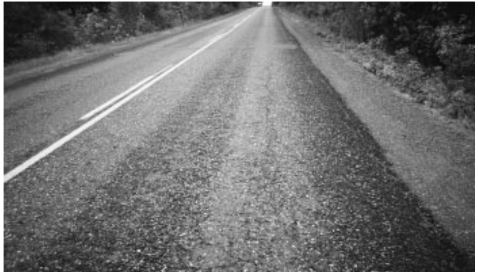
► Moderate to severe raveling in wheel paths.
