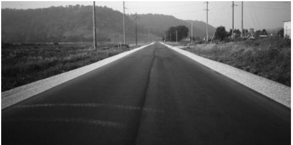
► RATING 9 Recent overlay, rural.
