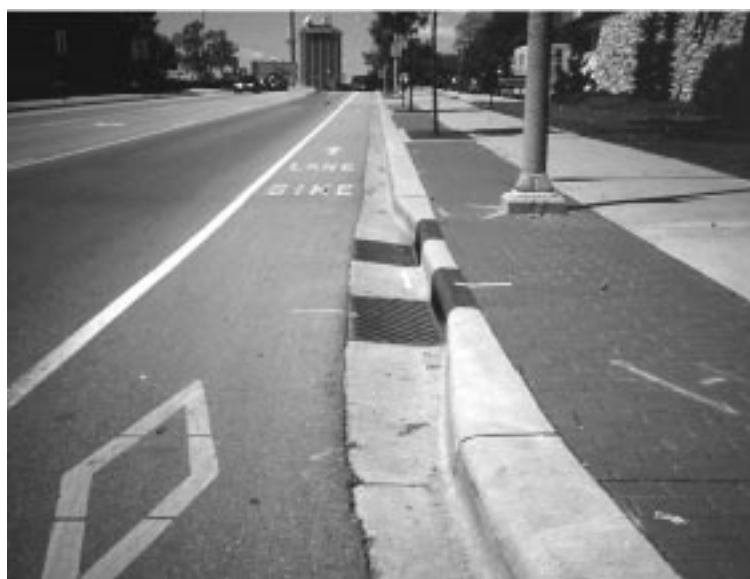
Urban drainage. RATING: Excellent
