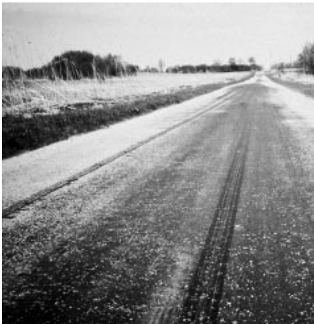
▼ Severe flushing.
