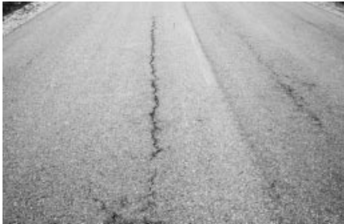
Multiple open cracks at center line, wheelpaths and lane center. ▼
