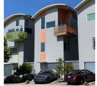
Figure 4.7 Example of what can happen without height standards calibrated to the existing context. These townhouses are “slot homes” that are out of scale with the existing context in terms of building height. They also fail to provide open space between units, making these less attractive to the consumer.
