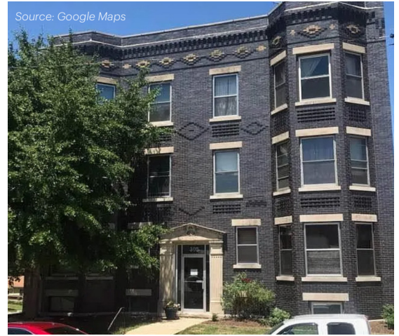
Multiplex 6 units - Gridley Allen Prickett Neighborhood
