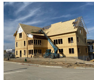
Figure 2.5 The simple forms, smaller size, and compatibility with simple wood-frame construction help maximize affordability and investment returns, and are consistent with the construction strategies familiar to most residential homebuilders, as shown in this under-construction MMH project in Papillion, Nebraska.
