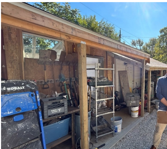
Figure 4. September 5, 2025, site inspection: Looking S from N side of covered walkway
