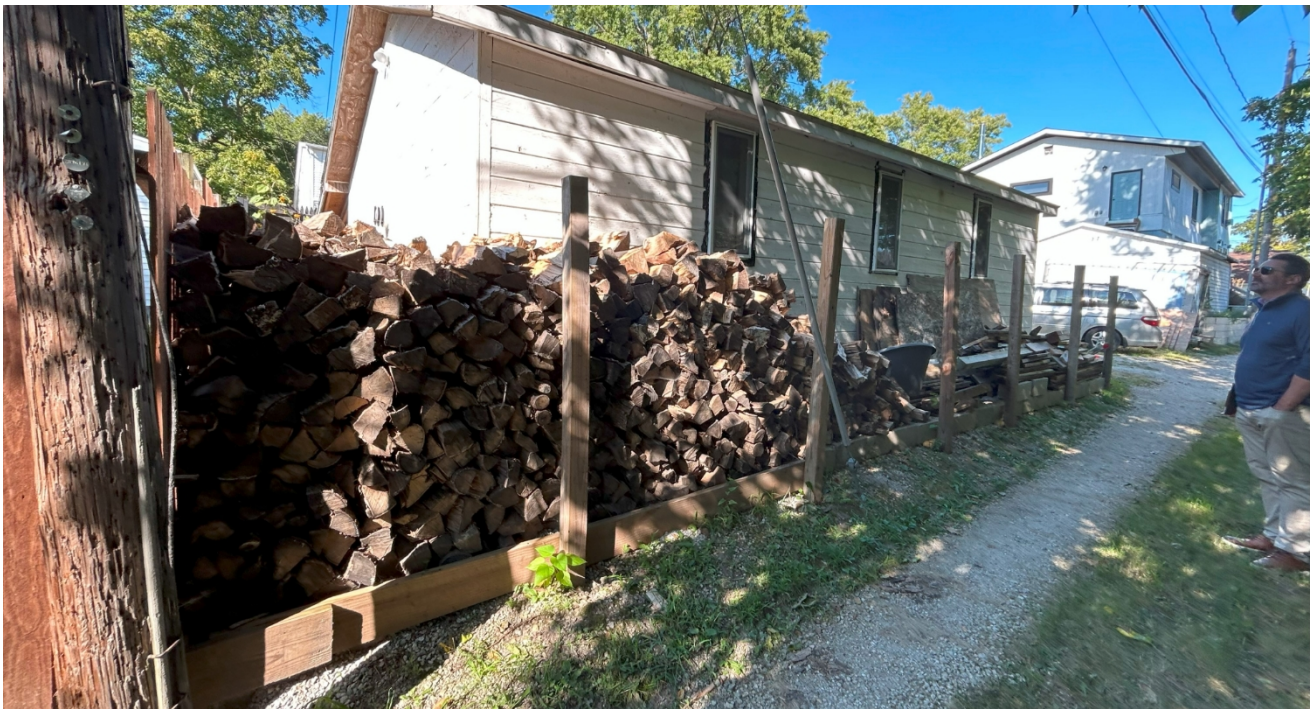
Figure 5. September 5, 2025, site inspection: Looking NE to S side of garage: note required yards filled with stacks of firewood.
