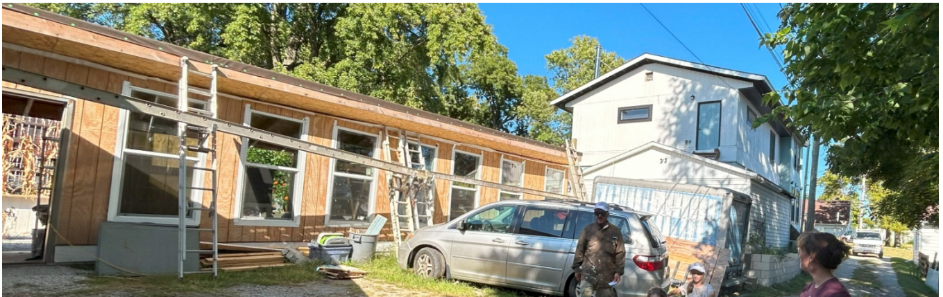
Figure 3. September 5, 2025, site inspection: Looking N from alley to south side of covered walkway.
