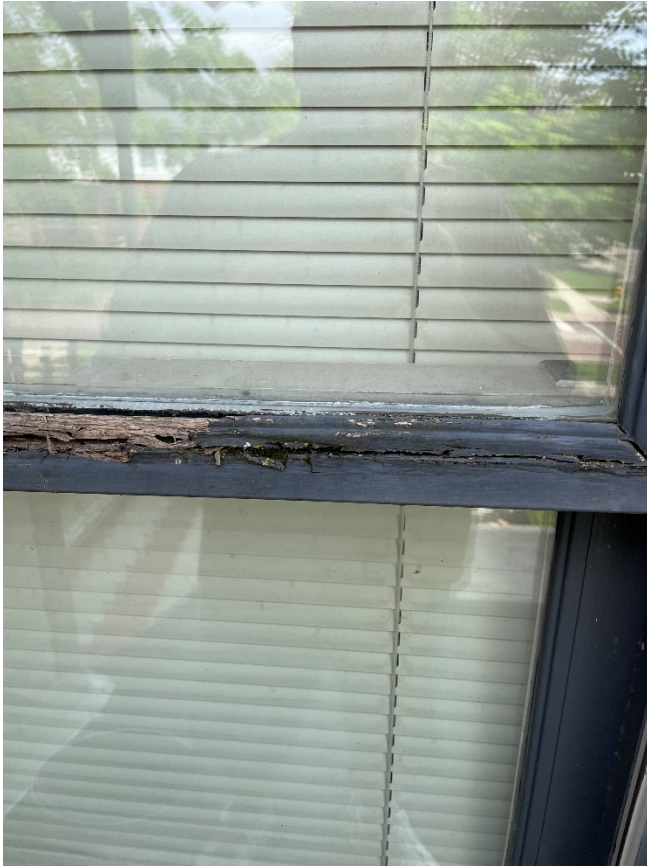
Attachment 1: Images of area where work is to be performed
