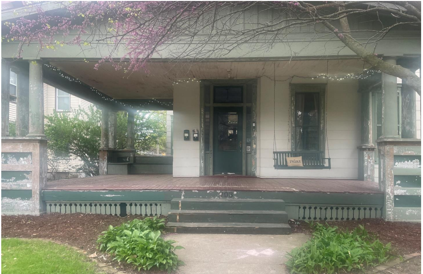
Attachment 1: Images of area where work is to be performed
