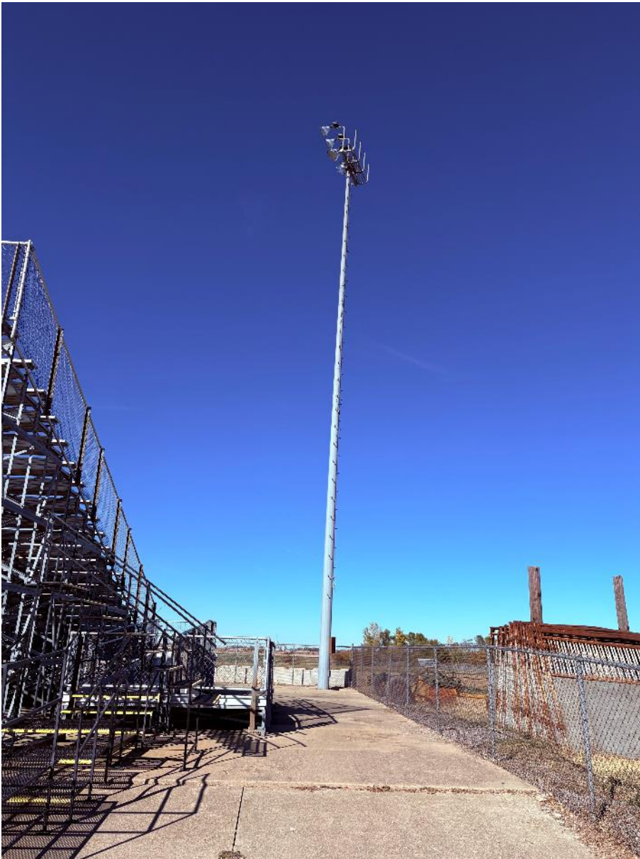
Figure 5. Looking north along track bleachers towards floodlight (left).
