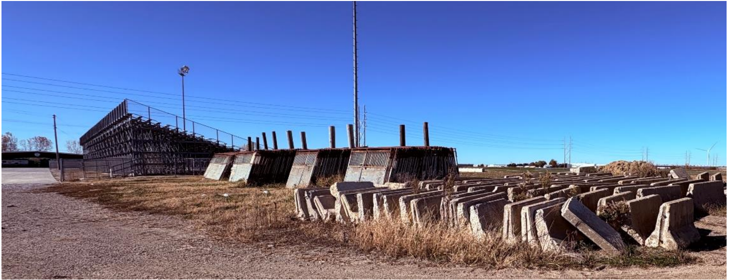
Figure 4. Looking west towards track with floodlights (above)..
